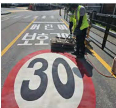
Road marking method (pre-formed fusion paint, story road)
